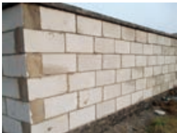
图5-16 粉煤灰砖砌墙
